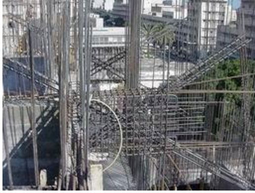
Fig. 7: The reinforcement arrangement of the core shear beams at construction.
