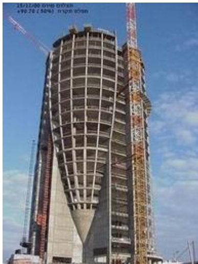
Fig. 3: The Eastern spatial wing at construction.
