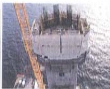
Climbing form for pylon legs
