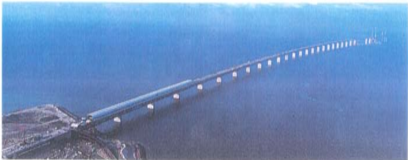
the approach bridge at Lernacken.
