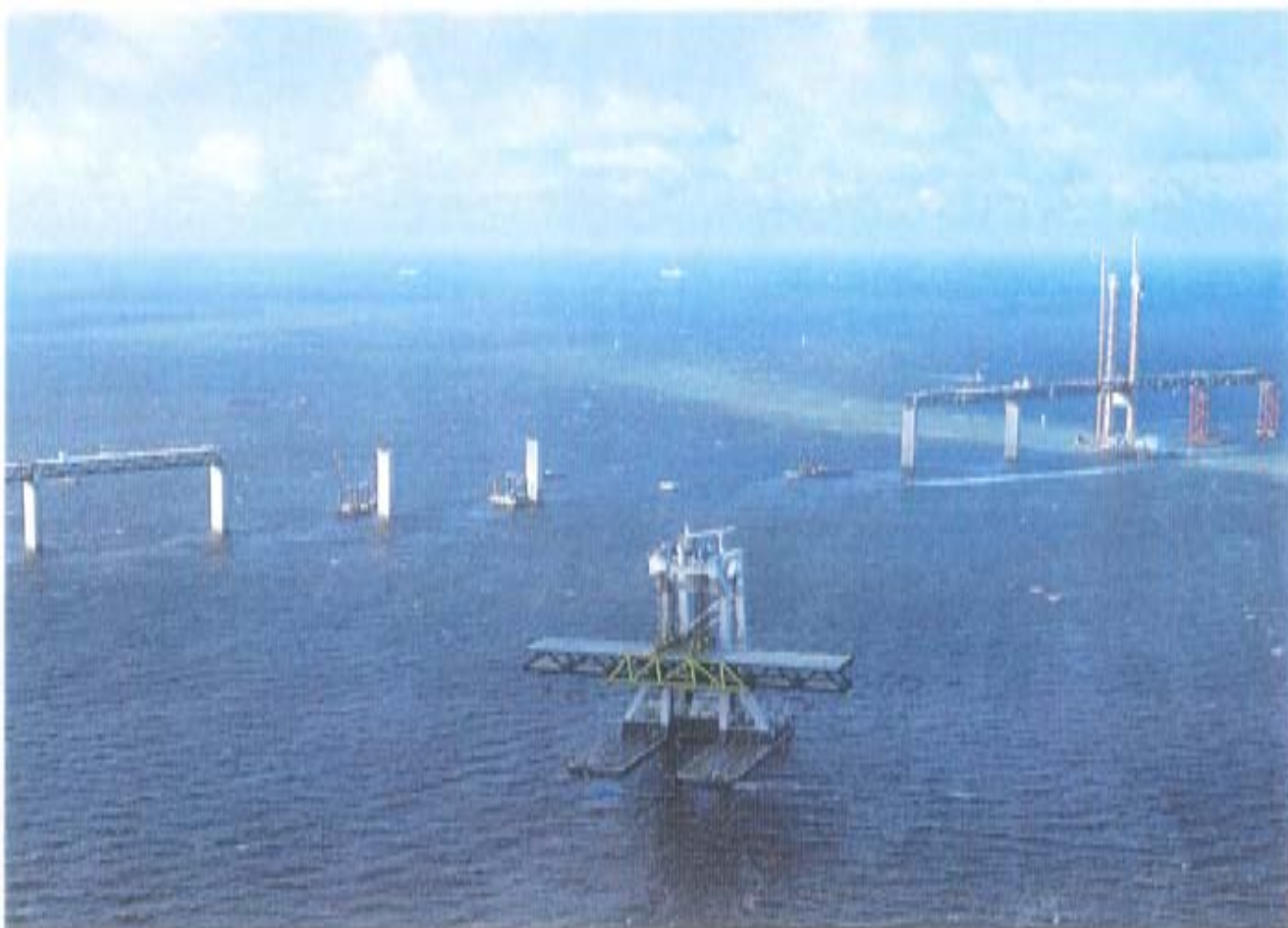
The floating crane "Svanen" places a bridge section in position.
