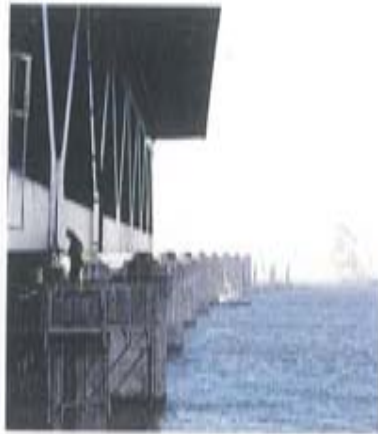
Work in the bridge line
