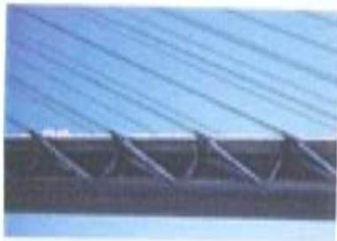
Cable anchorage brackets
