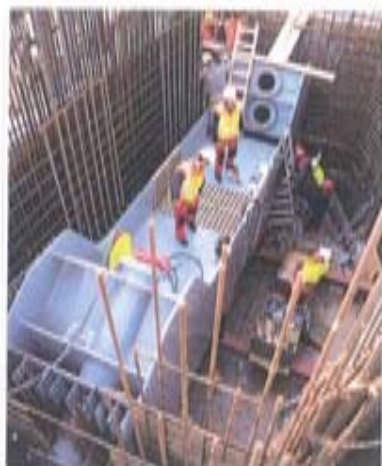
Installation of stay anchorage in pylon
