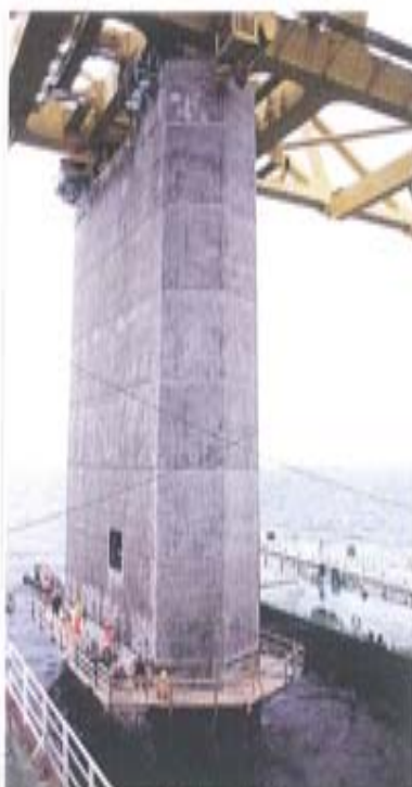
Installation of pier shaft
