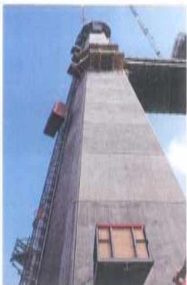
Pylon leg in in-situ concrete
