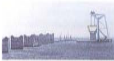
Svanen transporting pier shaft to the bridge line
